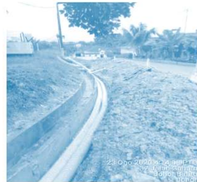
6 Inch HDPE Cable stretched
