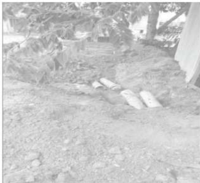
Joint pit is provided for cable jointing work
