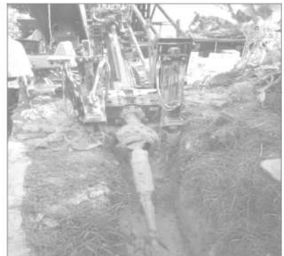
HDD Goodeng 32T Machine Used During Pipe Drilling Work
